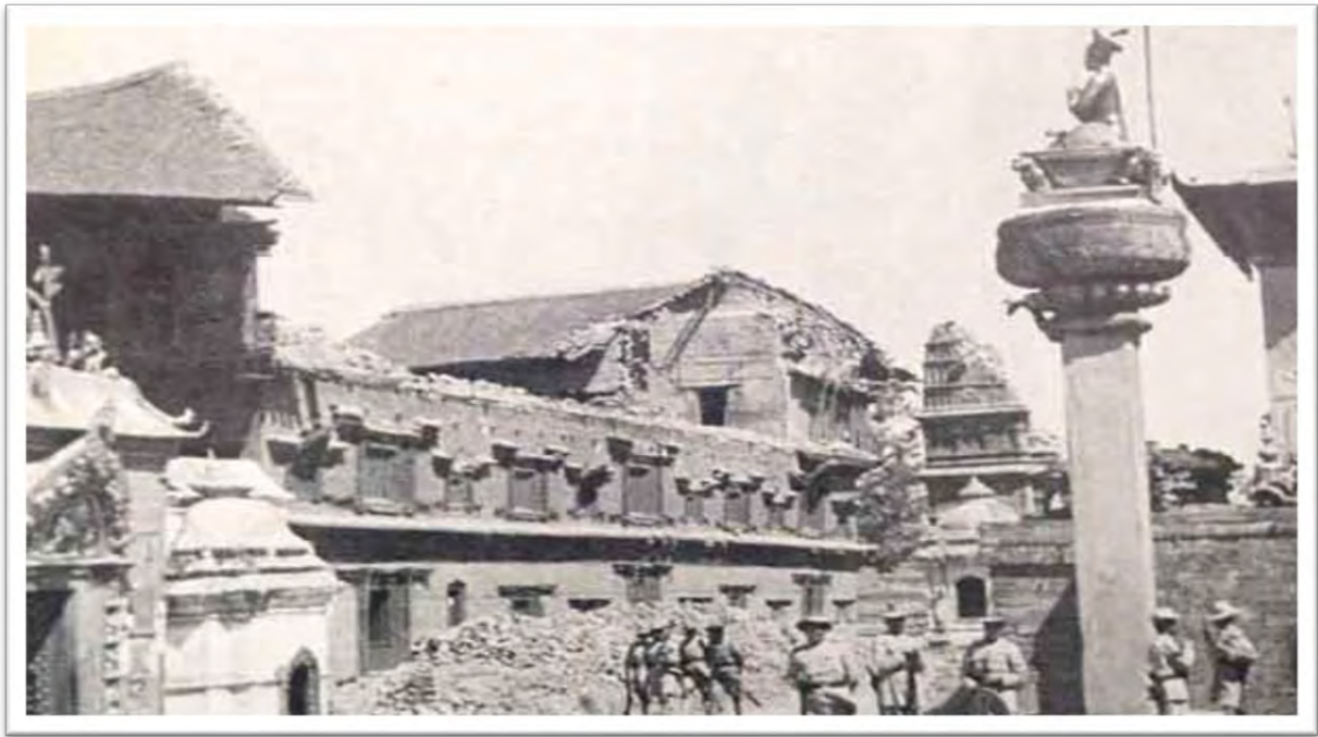
Temples of Nepal after earthquake in 1934 AD
